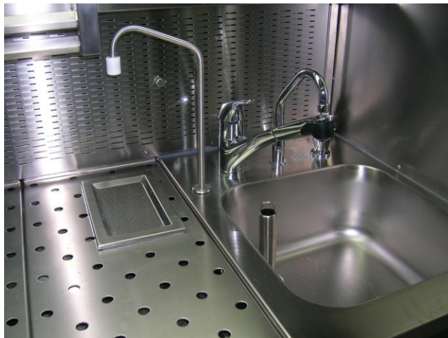
Fix installed Formalin Faucet with ball valve Typ: FZH-15-K
